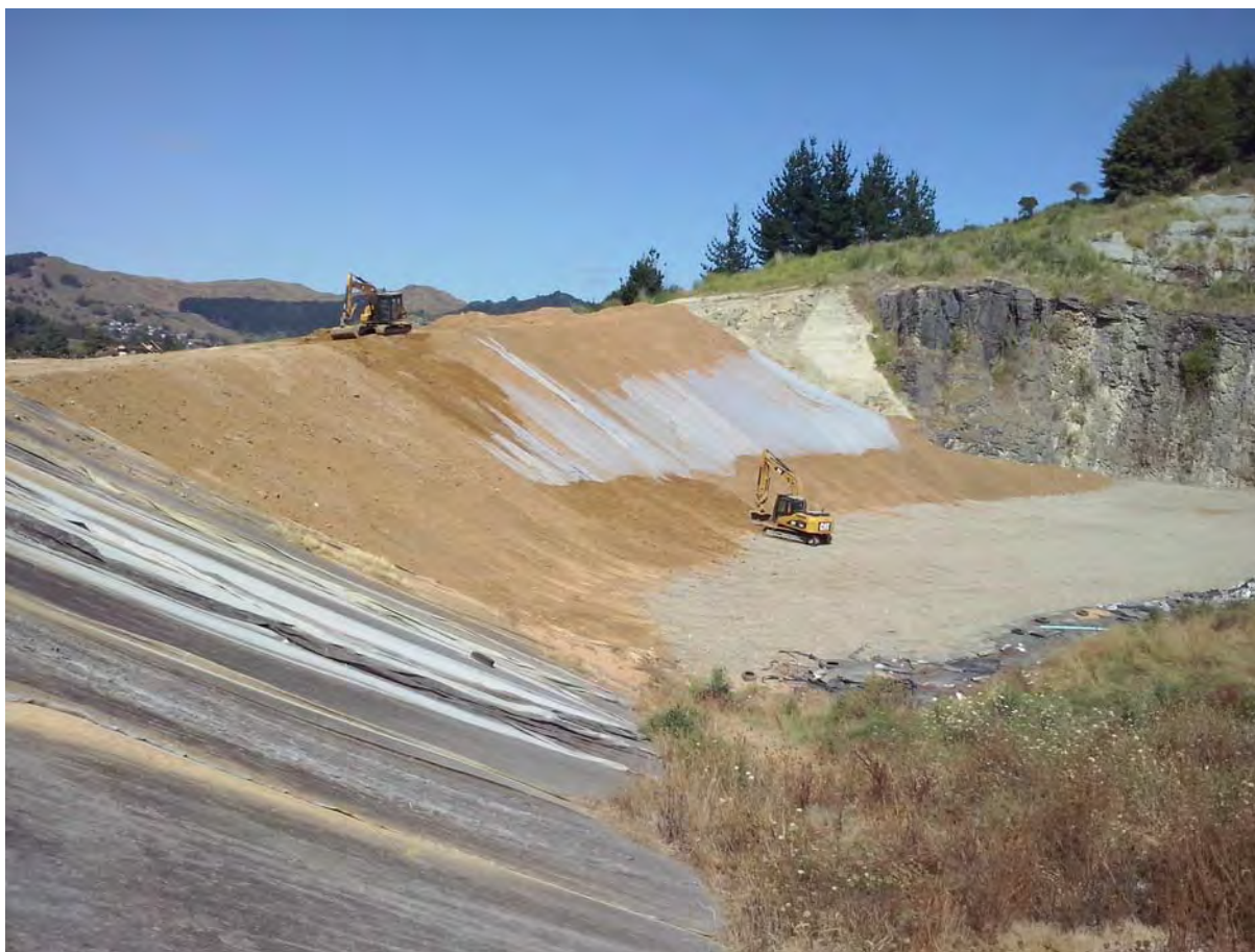
Cell 3 under development -2015
