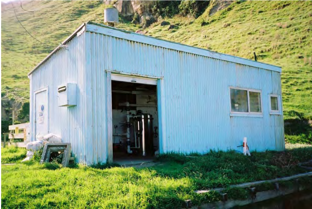
Mokau WTP building
