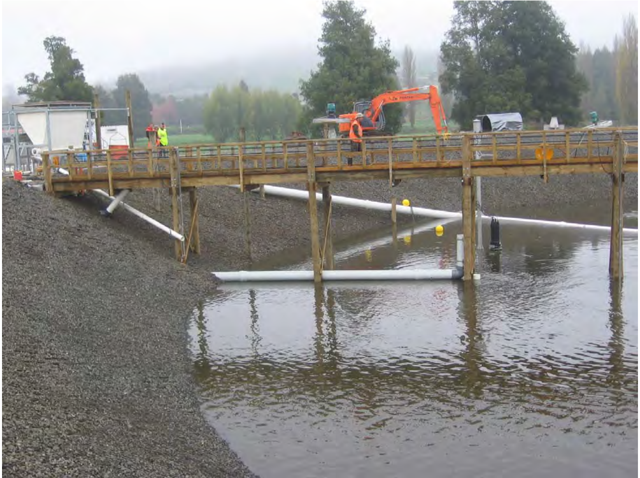
Fig. New Reactor April 2013
