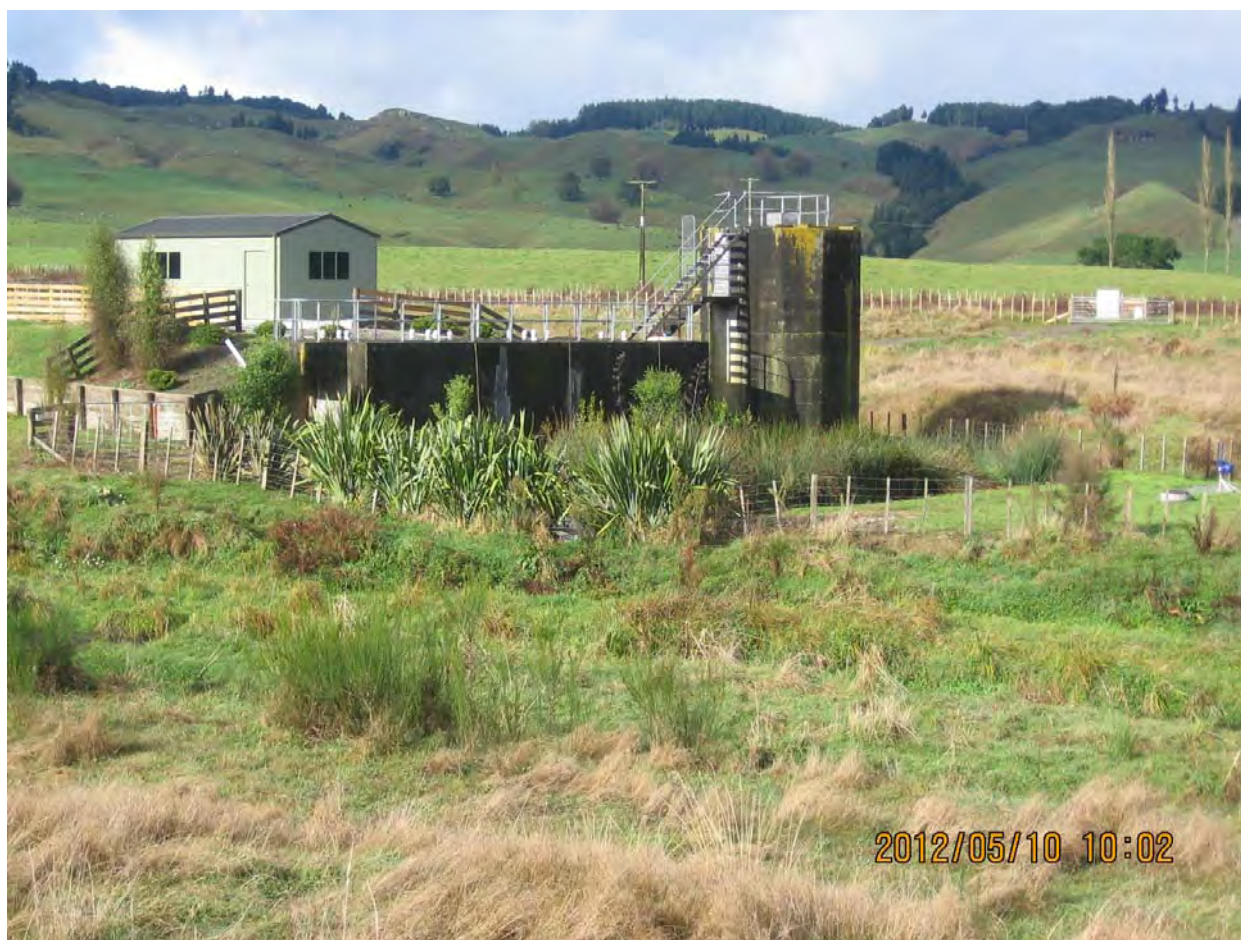
Benneydale Wastewater Treatment Plant
