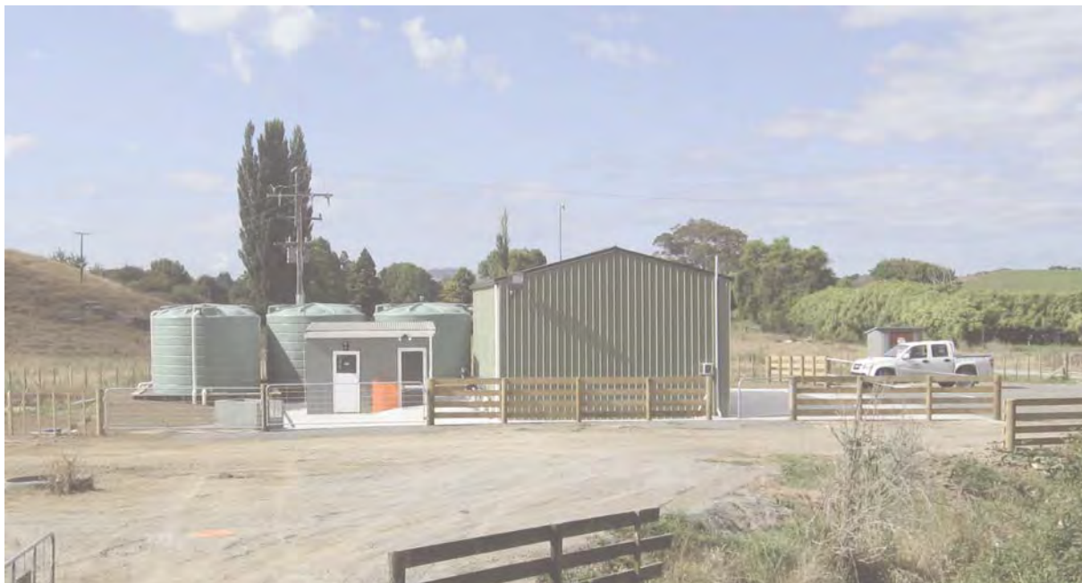
Fig.: New Piopio Water Treatment Plant
