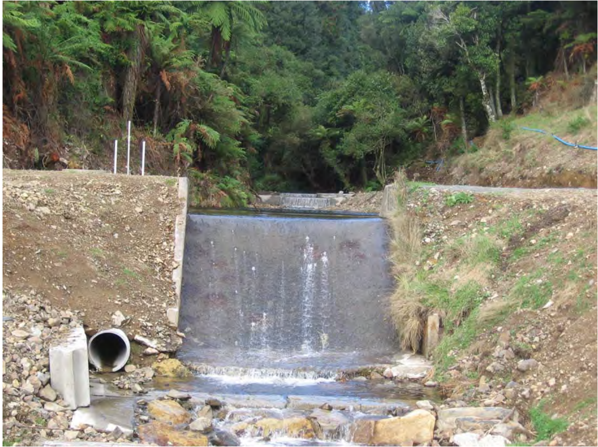
Fig.: Upgraded Intake spillway 2008 - Benneydale
