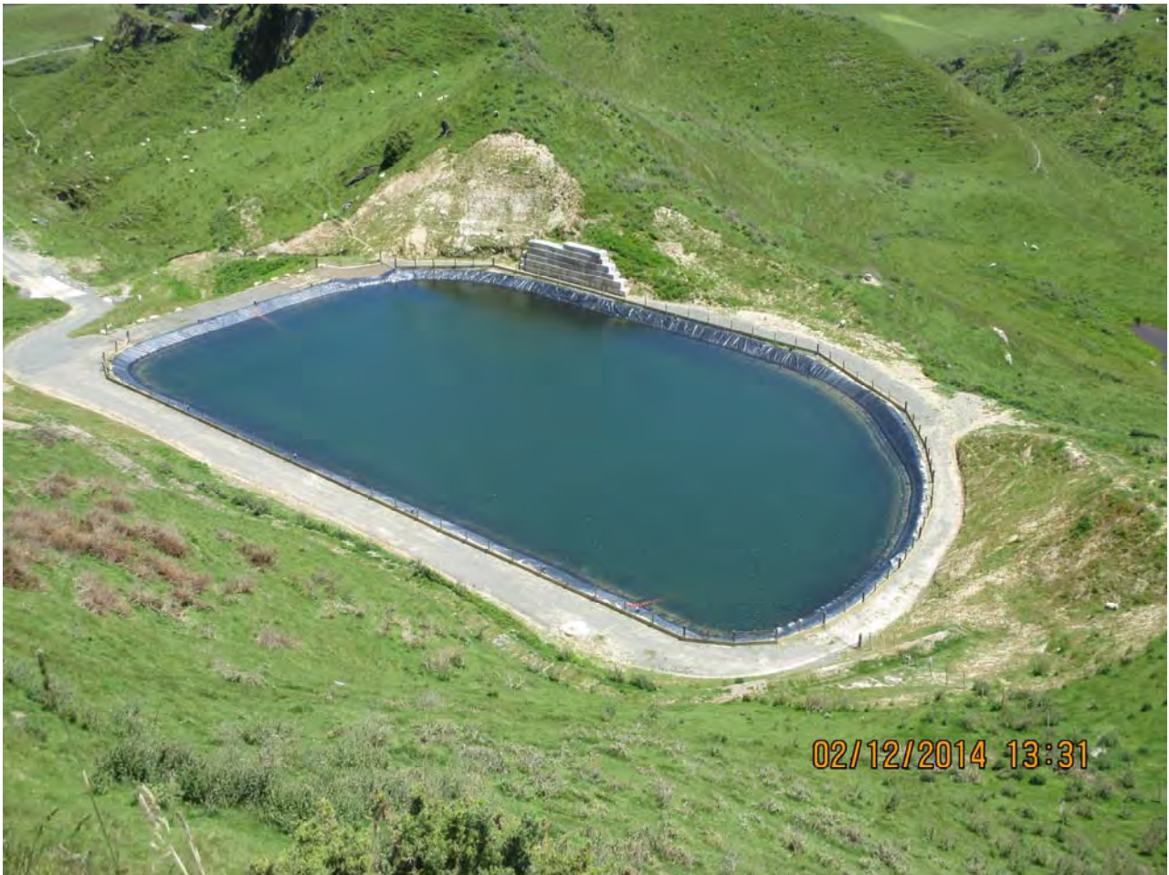
1Newly Completed Mokau Raw Water Supply Dam
